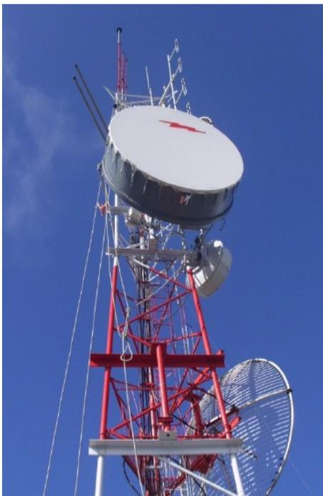
Figure 3. Frequency Diversity single antenna during installation at the lower site, Site B (1000 m AMSL), in Belize.
