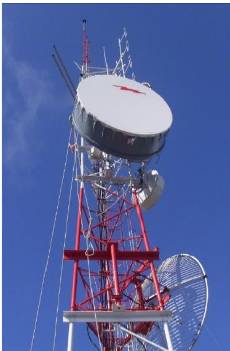
Figure 3. Frequency Diversity single antenna during installation at the lower site, Site B (1000 m AMSL), in Belize.
