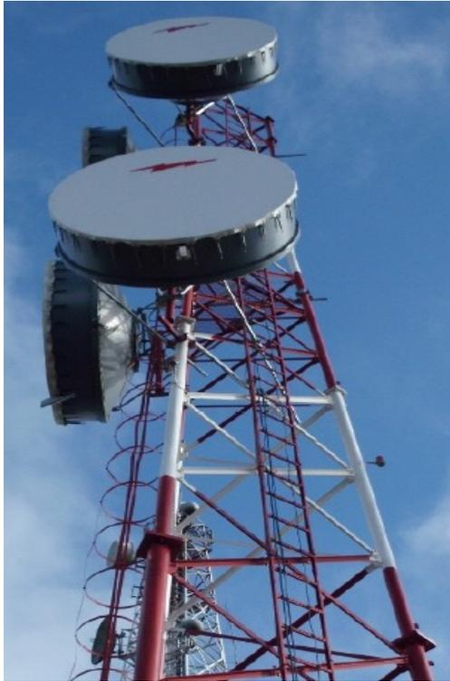
Figure 4. Frequency/Space Diversity in Honduras (1600 m AMSL) toward Site B. Note: The two antennas behind overlook a 193 km IP link over the Atlantic Ocean.
